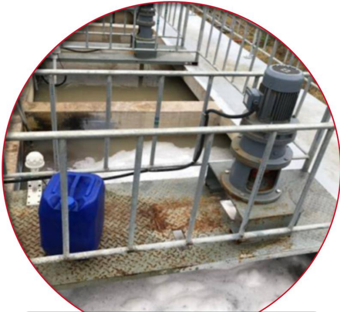
Privately owned wastewater treatment facilities
