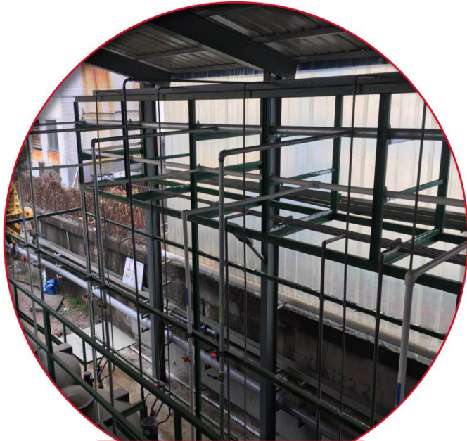
Water recycling facilities
